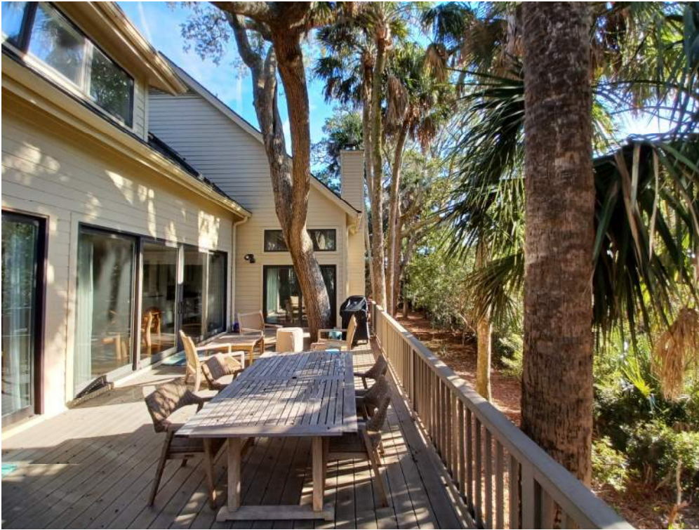
Rear view @ Deck level looking East
